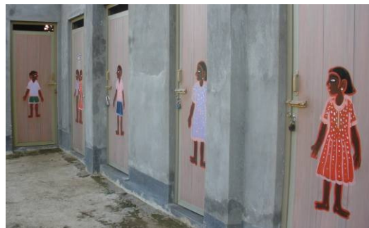
For the wonderful latrine block – now beautifully labelled – thanks again to Iiti Sydney
