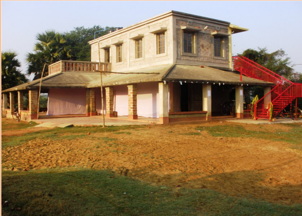
The completed upstairs – thanks to the trustees of the late Irene Breugel
